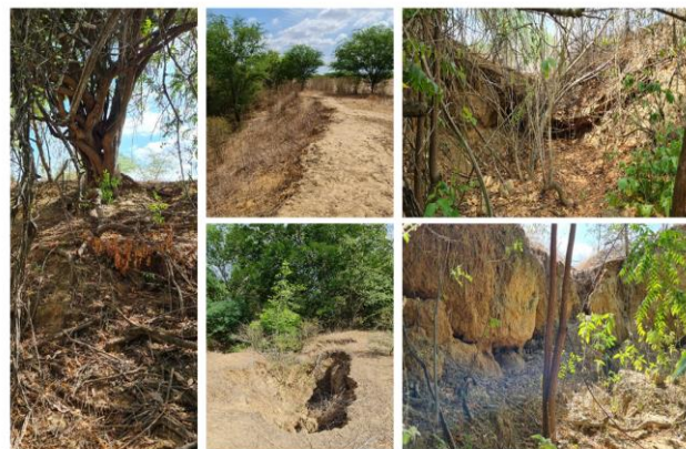
Figure 3 - Erosion processes in the vicinity of the Tapuio River, identified during the IV Scientific Expedition of the Lower São Francisco. Source: Nadjacleia Vilar Almeida e Milena Dutra (2021).
